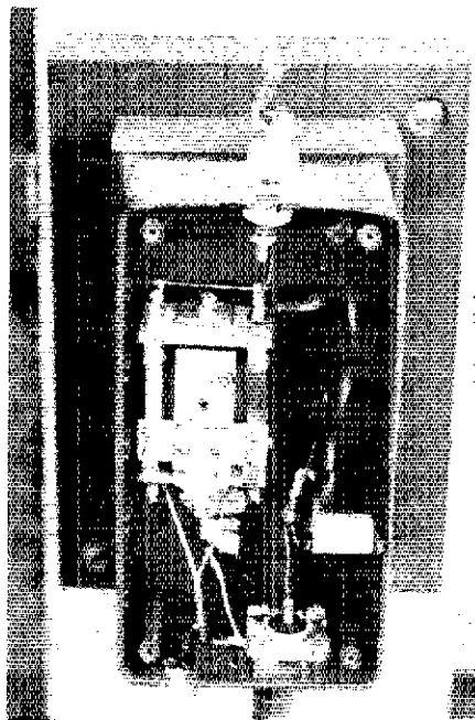
Fig 5—The feed-point enclosure for the dual-band inverted L at AE6C. Five high-voltage mica capacitors (at right) tune out the antenna's reactance at 80/75 meters.
